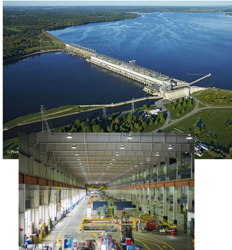
Carillon Generator station / Canada (14x 54 MW) Scope: re-equip turbine generator units and rehabilitation of hydraulic passage
