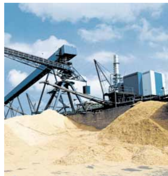
▲ ANDRITZ supplied a turnkey woodyard, including the first HHQ-Chipper™ in South Africa. The ECF bleach plant design is based on the mill's Bleaching Plant 3, delivered by ANDRITZ in 1994-1995. The new bleach plant has been operating at 1020 admt/d – already surpassing its design target.
