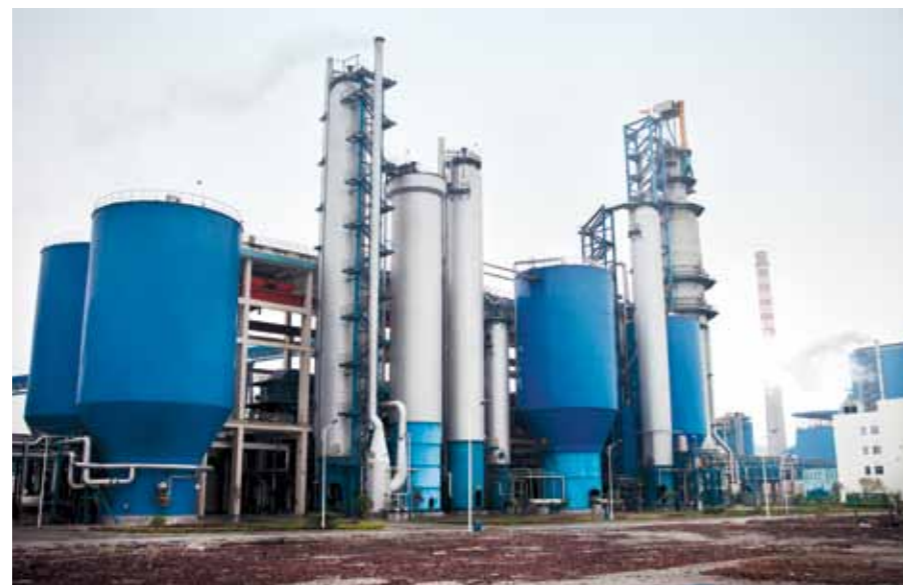
The fiberline at Huaihua is one of the largest in China. A total of six DD Washers are employed for washing, oxygen delignification, and ECF bleaching (left). Part of the oxygen stage and bleaching line. Bleached capacity is 1242 admt/d on softwood and 1358 admt/d on hardwood (right). ▼
