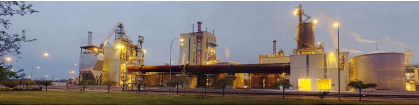
▲ The 8100 m 3 /d white liquor plant has a 600 t/d LMD kiln. "The X-Filters run great and the plant is very safe to operate," says Marcelo Garrido, Superintendent.
