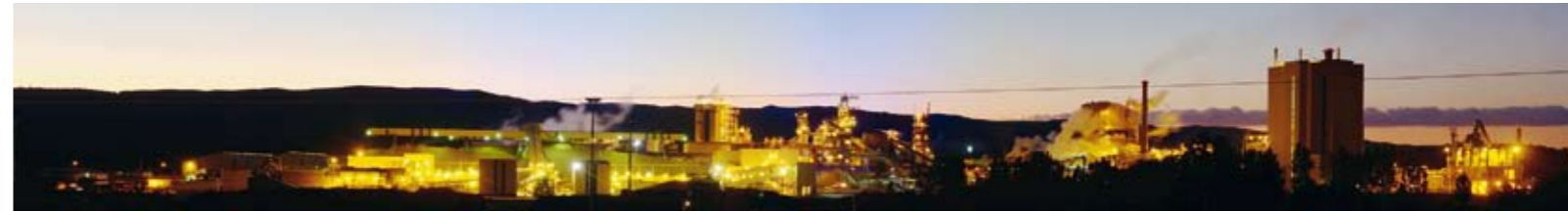
▼ Eucalyptus brownstock contains a high level of hexenuronic acids which consume chlorine dioxide in the bleach plant. Andritz’s patented A-Stage™ in the first bleaching stage reduces bleaching chemical consumption. There is also a large degree of filtrate recirculation in the bleach plant to minimize the effluent being discharged.
