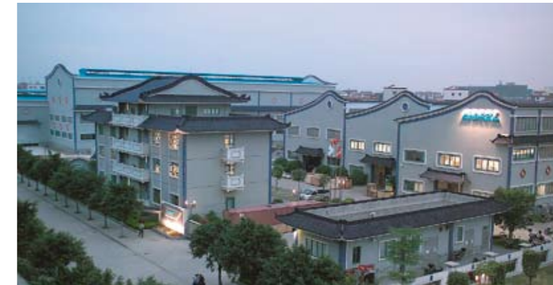
▲ A view of the Andritz Technologies Ltd. offices and plant near Foshan in South China.
