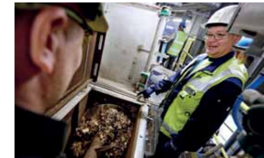
▲ Manne Koskinen, ANDRITZ Woodyard Technician, talks with an operator as they observe wood chips being fed to the BFB boiler.
