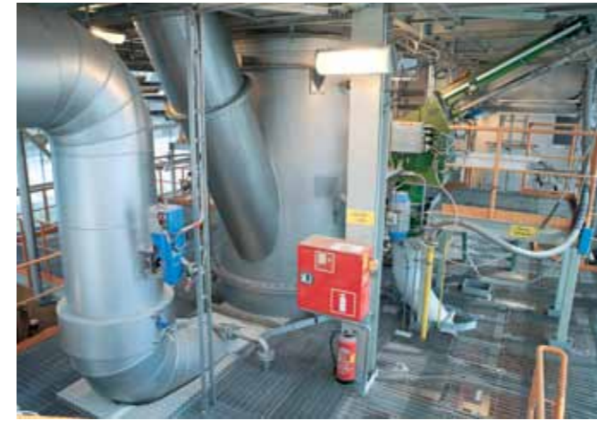
▲ Inside the CFB gasifier, which operates at about 750-800° C. The large duct on the left feeds air to the gasifier.
