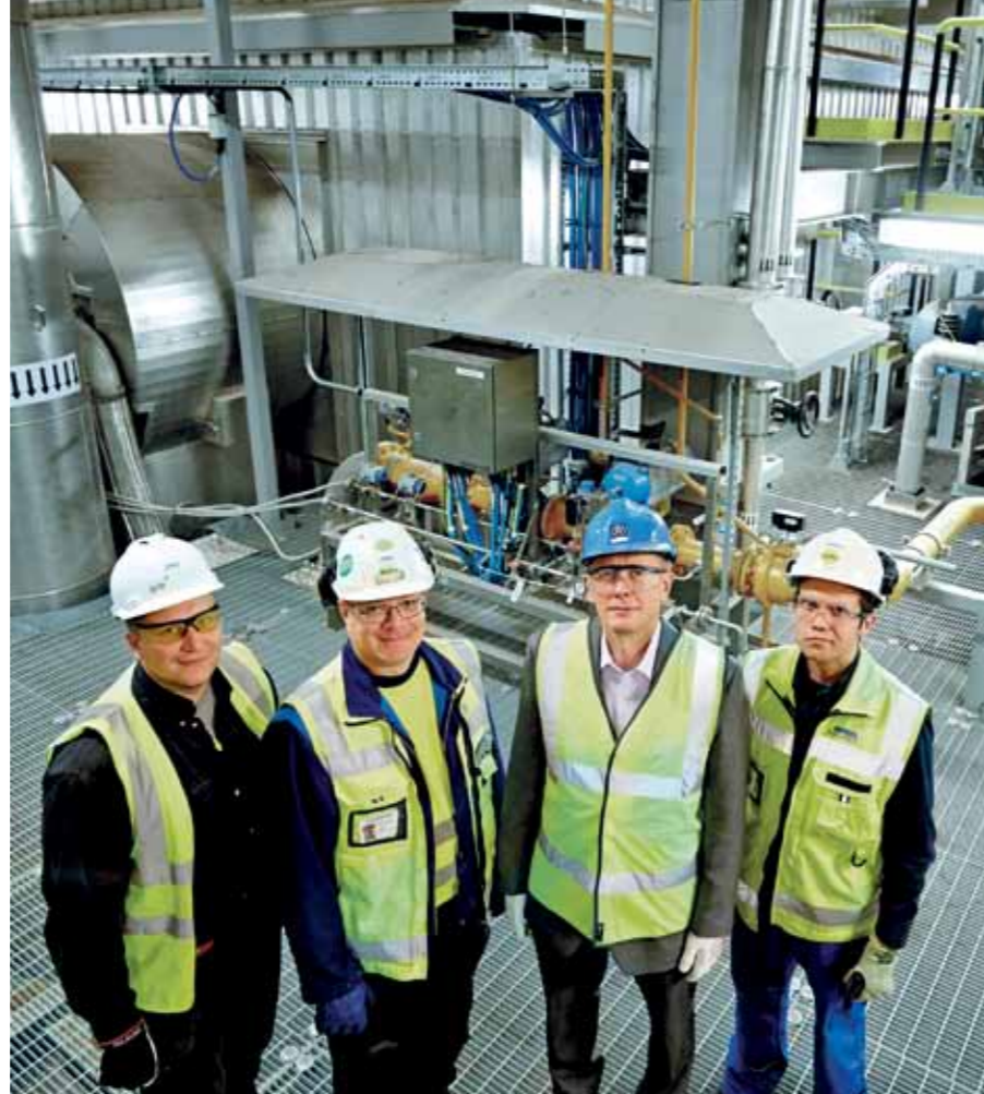
▲ (Left to right): Mikko Hänninen, ANDRITZ Boiler Commissioning Engineer; Manne Koskinen, ANDRITZ Woodyard Technician; Timo Nieminen, Workington's Power Plant Manager; and Ville Virtanen, ANDRITZ Commissioning Engineer in the boiler house.
