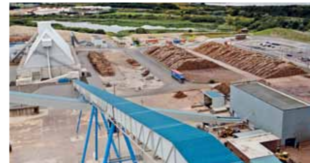
▲ ANDRITZ delivered the biomass receiving and handling system as part of the project. This included a chipping line for logs and a crushing line for wood waste. The A-frame building in the background stores 20,000 m 3 of biomass. The Workington Mill uses around 800,000 t/a of wood, mostly from Scotland and northern England.
