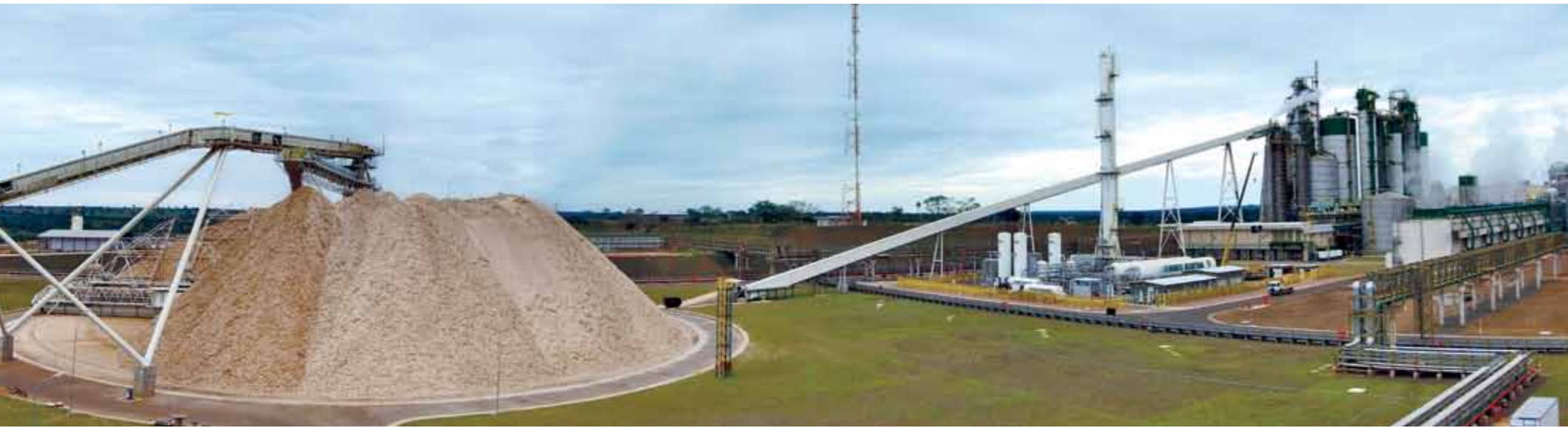
▲ View of the massive Eldorado mill from the woodyard. The new 360-degree Stacker-Reclaimer is in the foreground.
